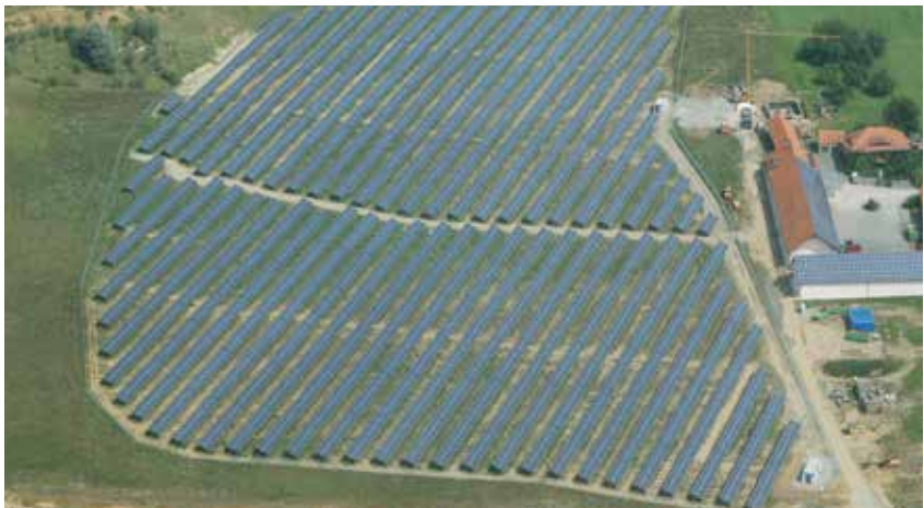
Mallersdorf-Pfaffenberg - Germany System: 3.463 MW | N-Rack System - Screw foundation
